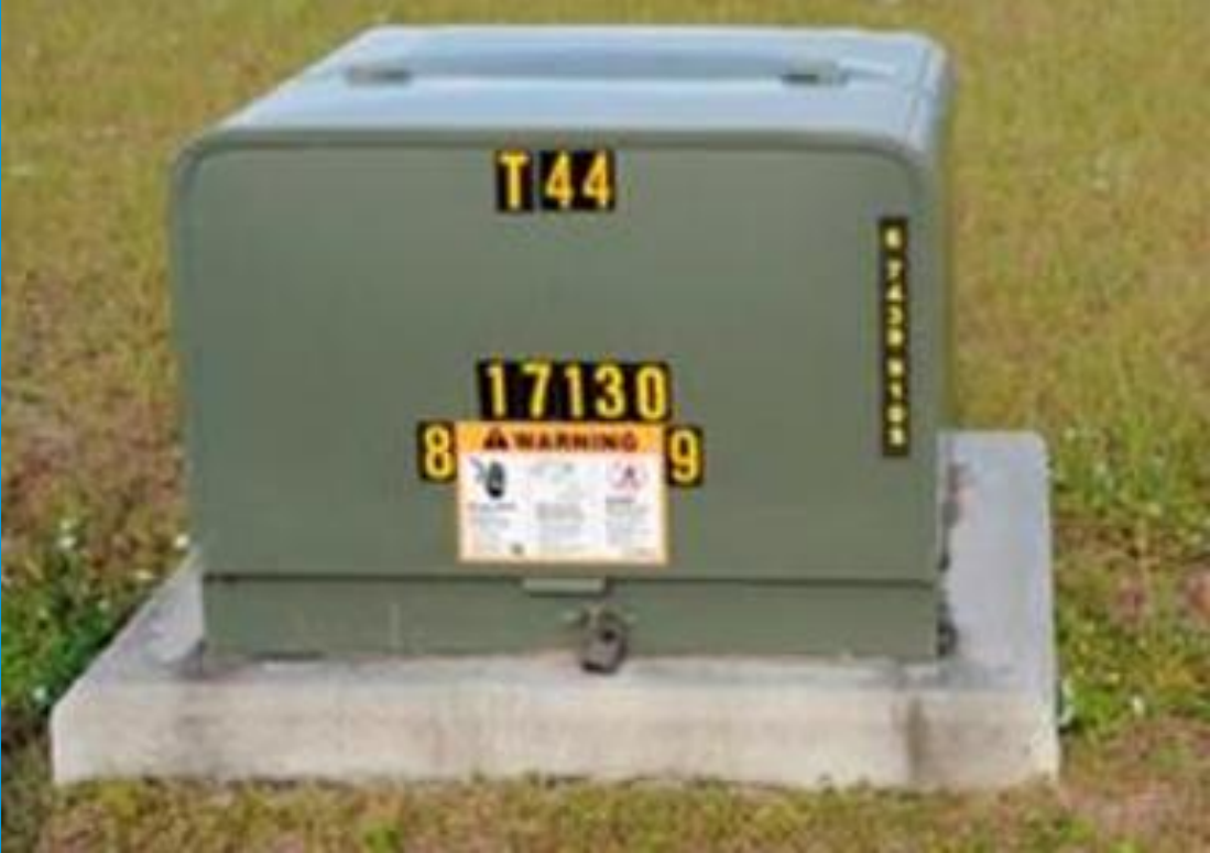
Pad-mounted transformer
