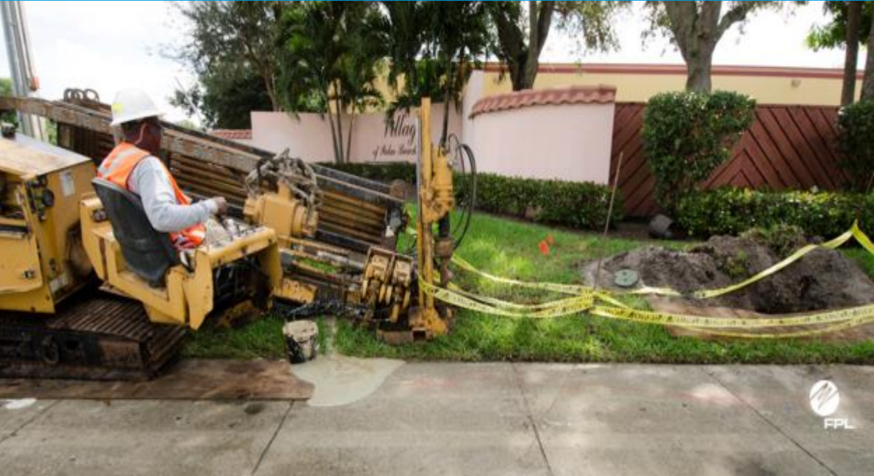
Horizontal or directional boring equipment
